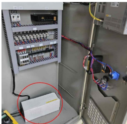
UPS Device Installation
